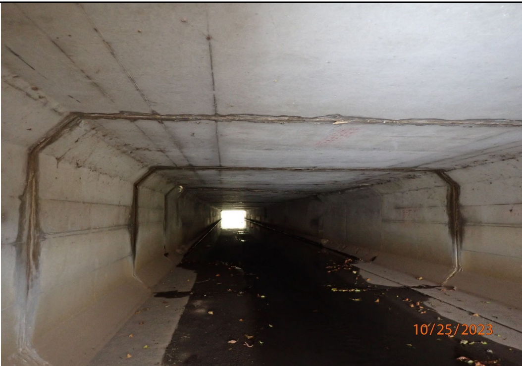
MP 417.63_CIN 41763011XX_CulvertInterior_PrecastExtension
